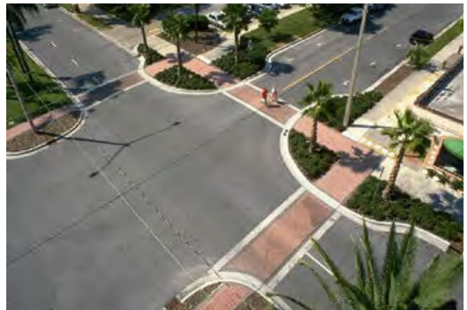
A pedestrian friendly example of curb extensions that can help slow down traffic and reduce crossing distances.
