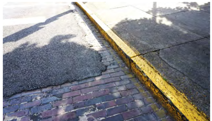
Old meets new - Bricks with granite curbs
