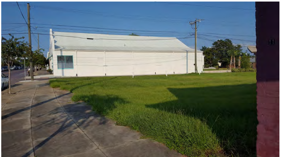
Temporary Interventions: Existing Conditions
